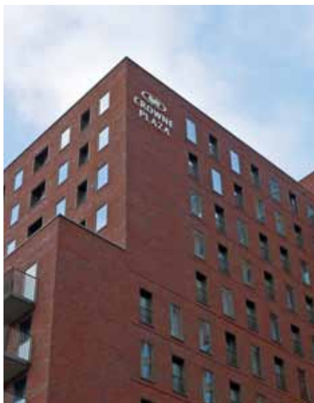
Crowne Plaza Hotel project
