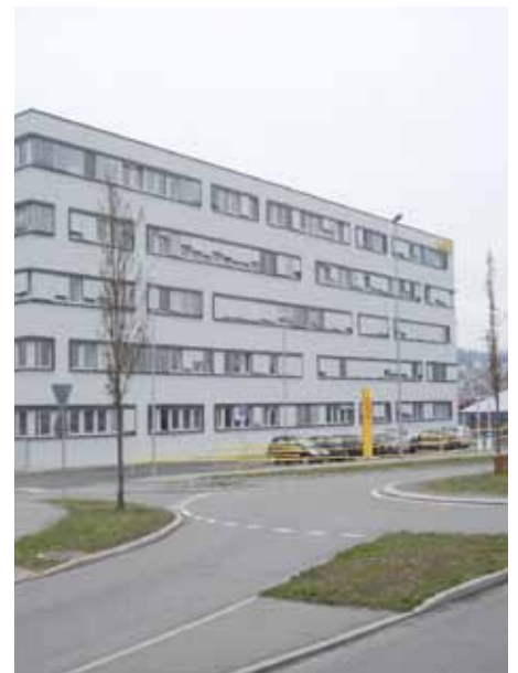
Logistics Centre, Regensdorf
