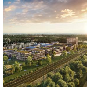
Timber Factory, Munich Site: 29,000m 2 Completion: 2027
