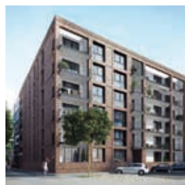
The Brick, Hamburg Apartments: 101
