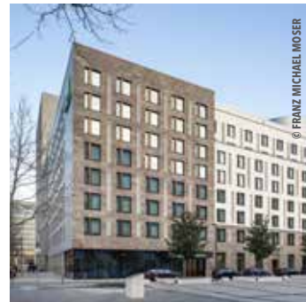
City hotel Holiday Inn Alte Oper, Frankfurt Rooms: 249
